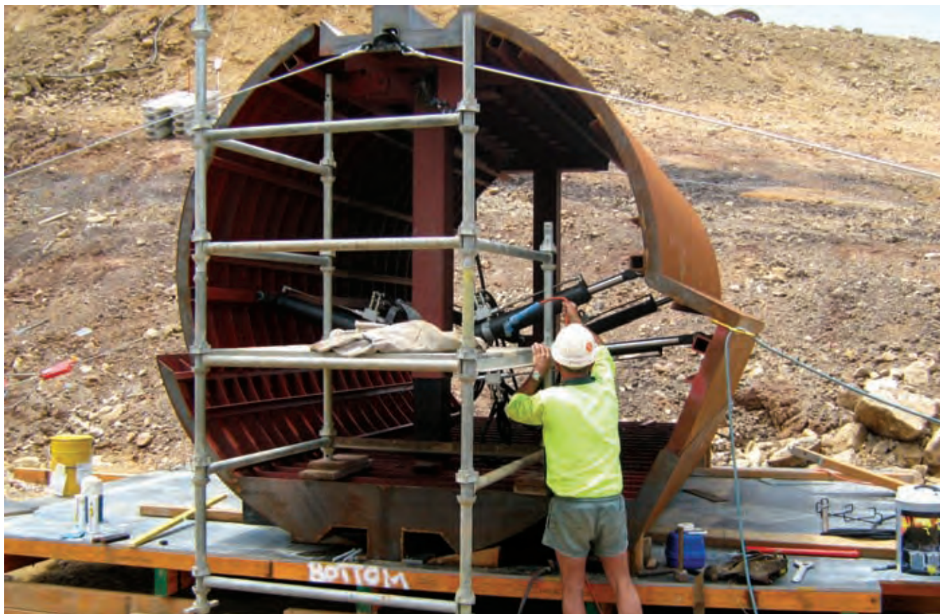
The intake tower formwork arrives onsite at Shannon Creek.
